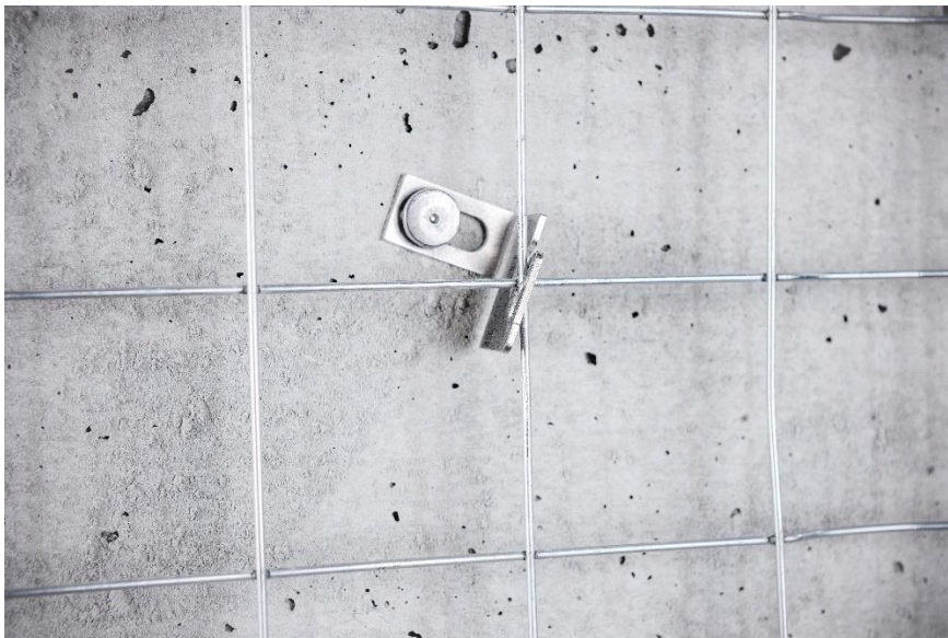
Fastening of light wire mesh reinforcement for fire protection mortar
