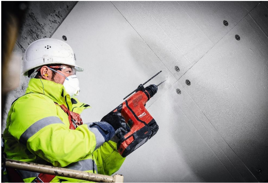
Fastening of pre-fabricated fire protection boards
