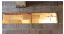
Large blank openings
